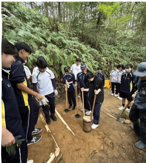
Repairing the road called "Michibushin"
